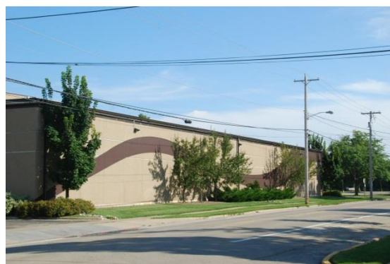
Neenah Water Filtration Plant
